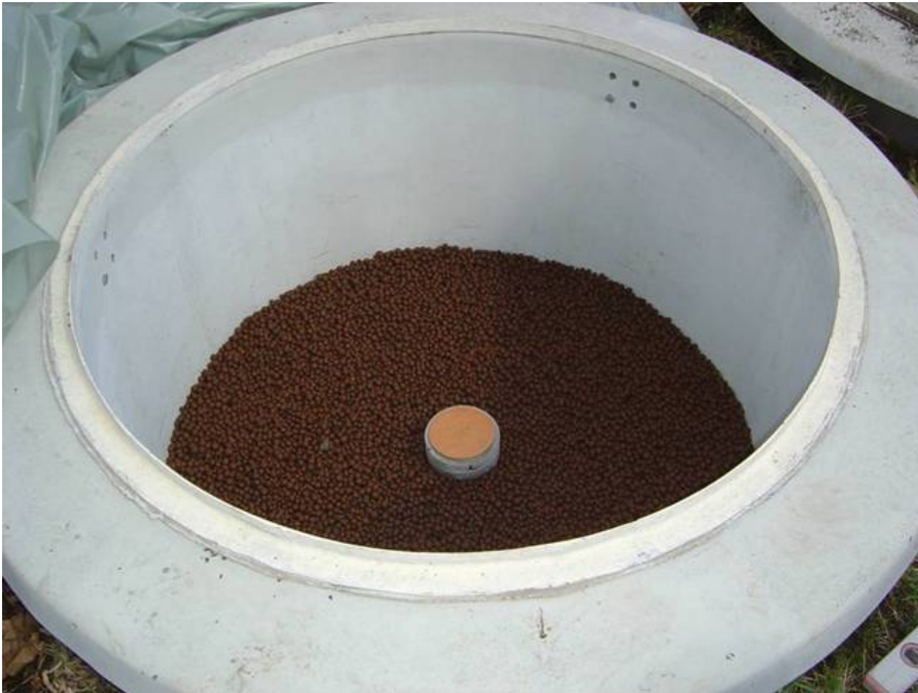
View on water drain and extended clay
