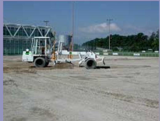
Construction of the sub base with crushed stone aggregates
