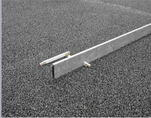
Evenness check of asphalt mortar and level corrections
