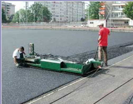
Elastic layer constructed in situ
