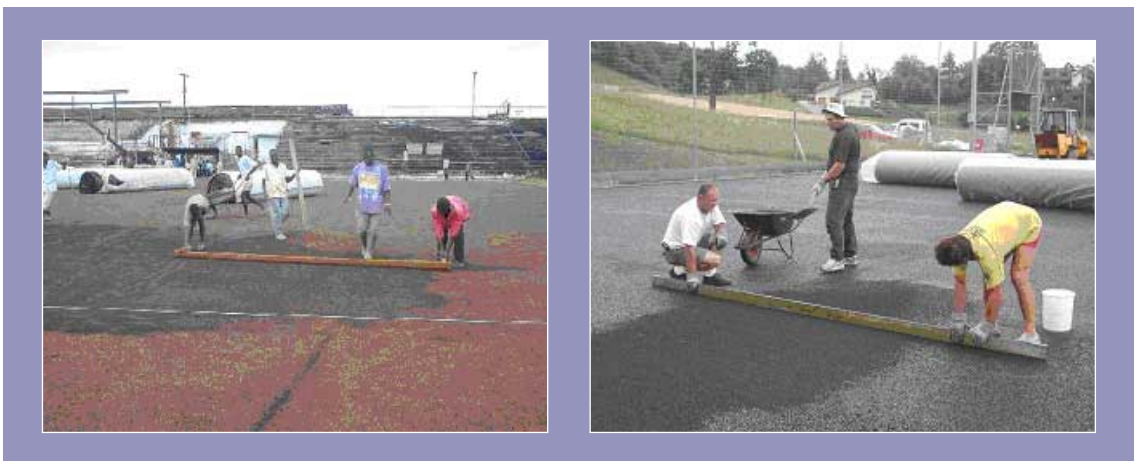
Fine levelling of a non-stabilised sub base and a bitumen stabilised finish
