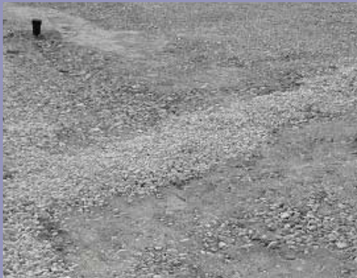
Construction of the sub base with crushed stone aggregates
