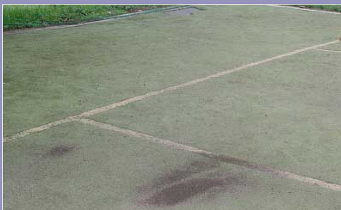
Artificial turf installed on unstabilised infrastructure
