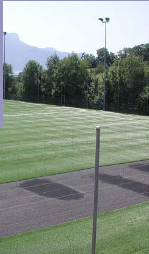
Minor level corrections on a 14-year-old elastic layer prior of the laying of a new turf.
