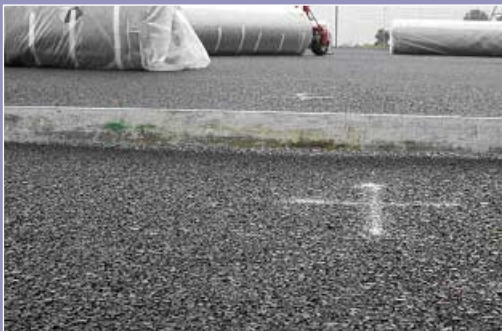
Deformation of the infrastructure
