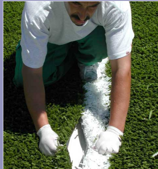
Gluing the joints and line markings
