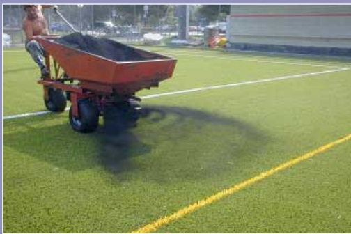
Filling the turf with sand and rubber granules
