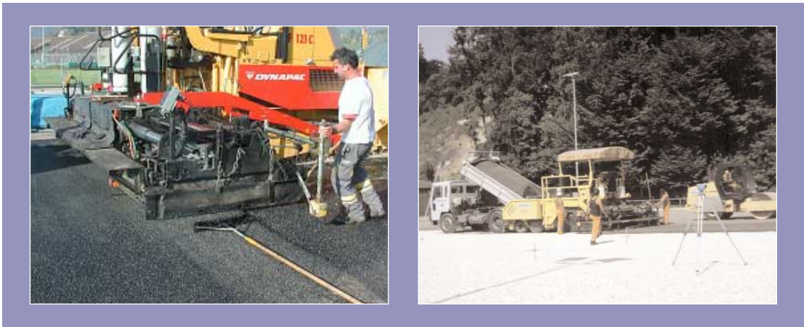
Laying of the asphalt binder course with electronic control levelling device
