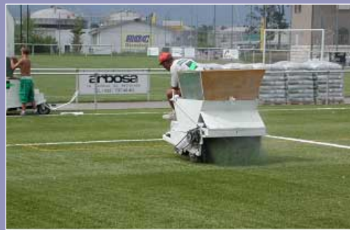
Stabilisation infill with quartz sand
