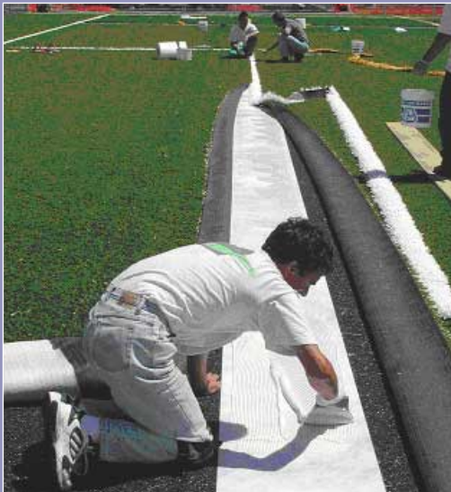
Gluing the joints and line markings
