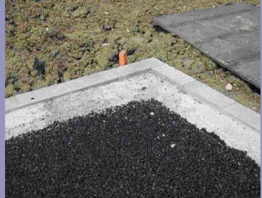
Curb stones as edging for artificial turf
