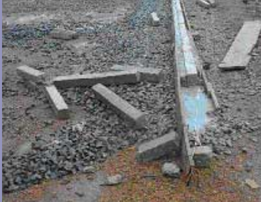
Curb stones as edging for artificial turf
