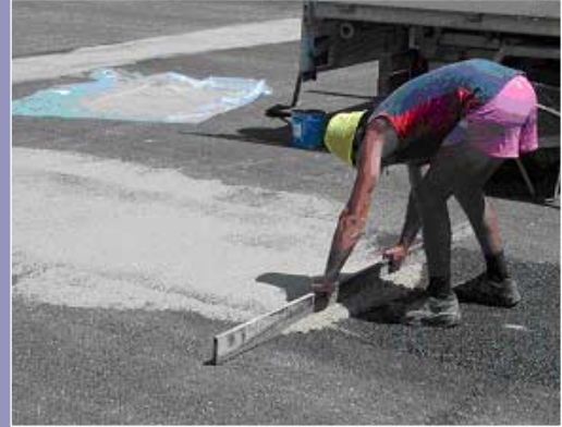
Evenness check of asphalt mortar and level corrections
